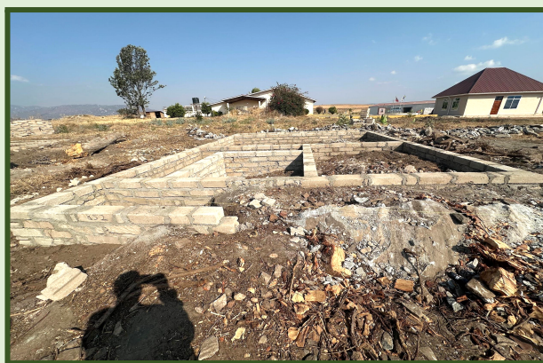
Foundation for the future cabins and social hall
